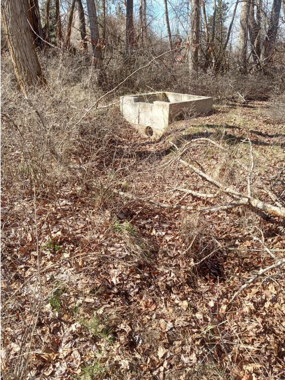
Photo A4 - Photo of Ditch 1 control valve bunker, facing east up Ditch 1. Note lack of bed material sorting or cut bank, and leaf litter.
